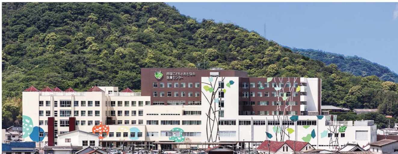
東側外観 View from east
